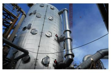
Stainless steel converters using flat bed support plates and divider plates welded to the shell, which basically copy the old carbon steel design, have experienced failures as a result of the differential rate of thermal expansion of the plate and the shell during heat-up.
